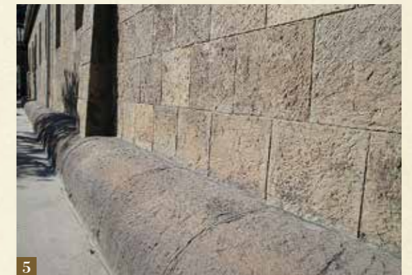
5 Chisel marks can be seen on the carefully stacked stones. The Japanese architectural style called 'Kamebaraishi' can also be seen at the building's foundation.
