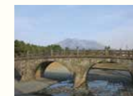
Stone bridge masonry techniques (Nishida Bridge)
