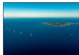
Block Island Wind Farm
