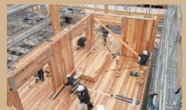
●CLT panel construction method
