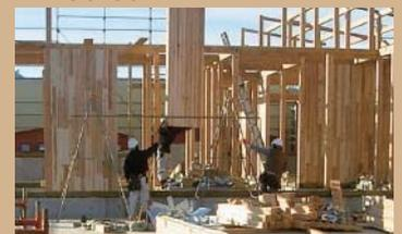
●Wooden frame + CLT construction
