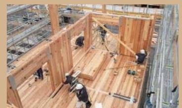
●CLT panel construction method
